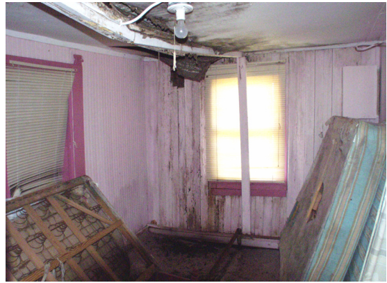
Figure 40 View to west in Room 104. (NPS-SERO-CR, 2002)
