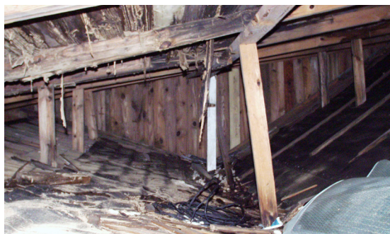
Figure 26 View of junction of roofs of two original structures; note severe termite damage in rafters and decking at left. (NPS-SERO-CR, 2002)
