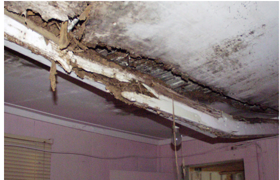
Figure 41 View to east of ceiling in Room 104. (NPS-SERO-CR, 2002)
