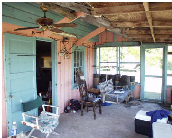
Figure 31 View to north on front porch. (NPS-SERO-CR, 2002)
