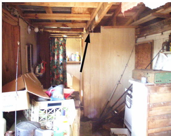
Figure 42 View northwest in Room 105. Arrow marks header at outside of historic porch. (NPS-SERO-CR, 2002)
