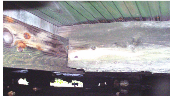
Figure 24 View of typical joist sill connection. (NPS-SERO-CR, 2002)
