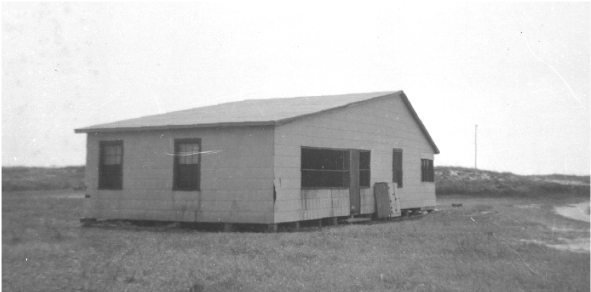
Figure 18 View to east of Lewis-Davis House in August 1958. (CALO Coll.)
