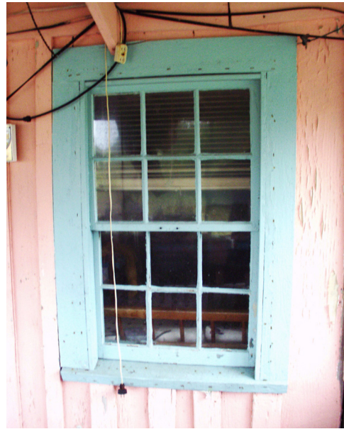
Figure 29 View of window W-2 on southeast (front) side of house, with exterior siding and trim typical of the original building. (NPS-SERO-CR, 2002)
