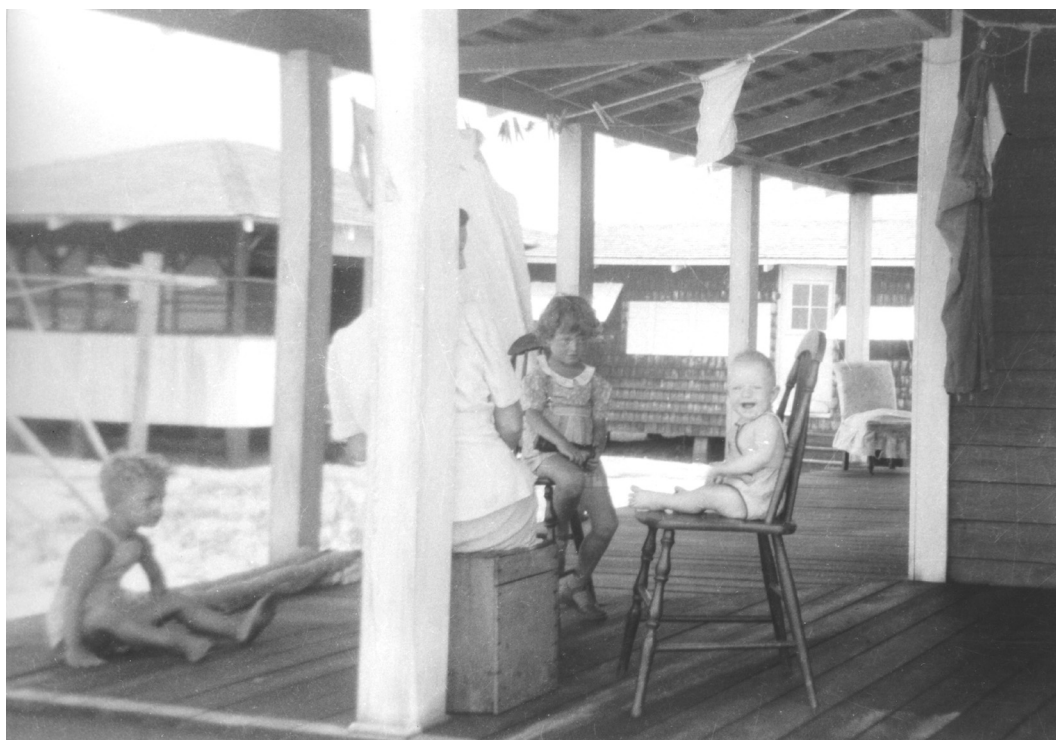
Figure 12 View of porch of Carrie Davis' store, October 1942. The dance hall is at left rear and her shingled house at center rear. (CALO Coll., Royer photographs)
