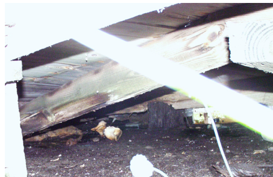
Figure 25 View of collapsing floor under Room 104. (NPS-SERO-CR, 2002)
