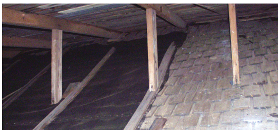
Figure 27 View of wood shingle roof on original structure encompassing Rooms 100 and 101. (NPS-SERO-CR, 2002)
