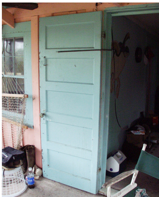
Figure 30 View of front door D-1. (NPS-SERO-CR, 2002)
