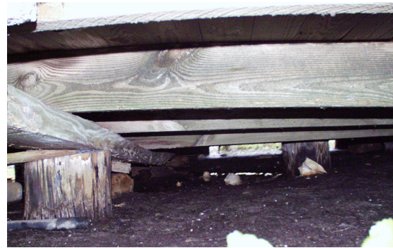
Figure 23 View of crawl space and piers. (NPS-SERO-CR, 2002)
